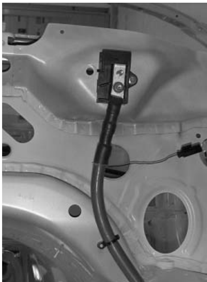
Cable Routing on Firewall
